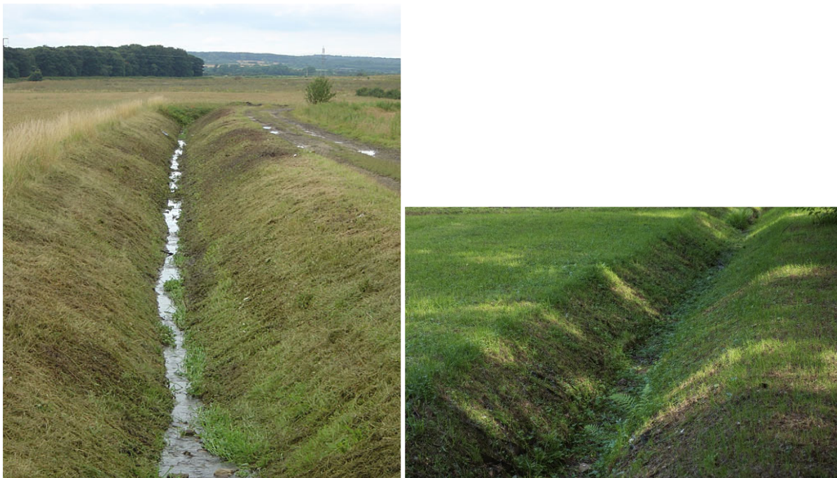
Figures 5&6. Typical examples of a V-shaped drainage ditch
